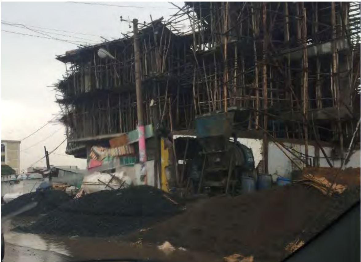
Fig.2.5 Fine and Coarse Aggregates stored aside roads
