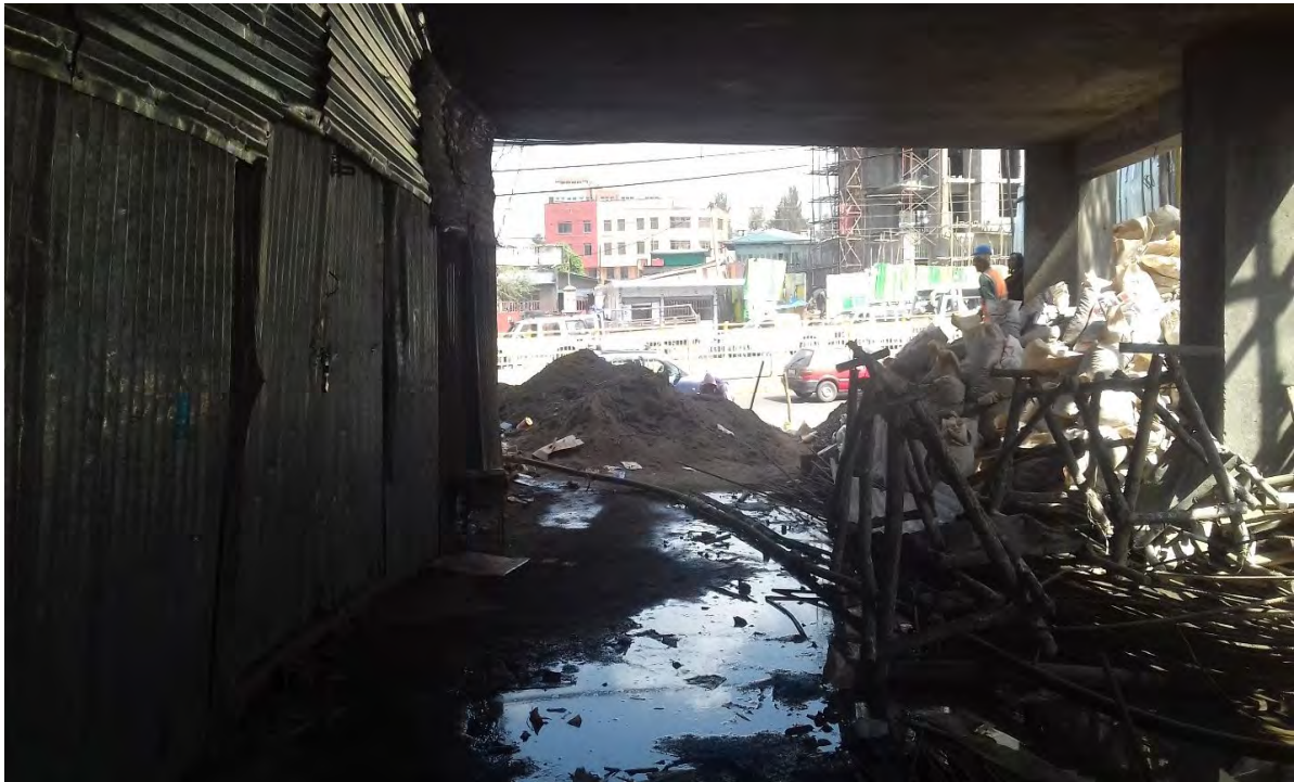
Fig.4.3: limited storage area on site
