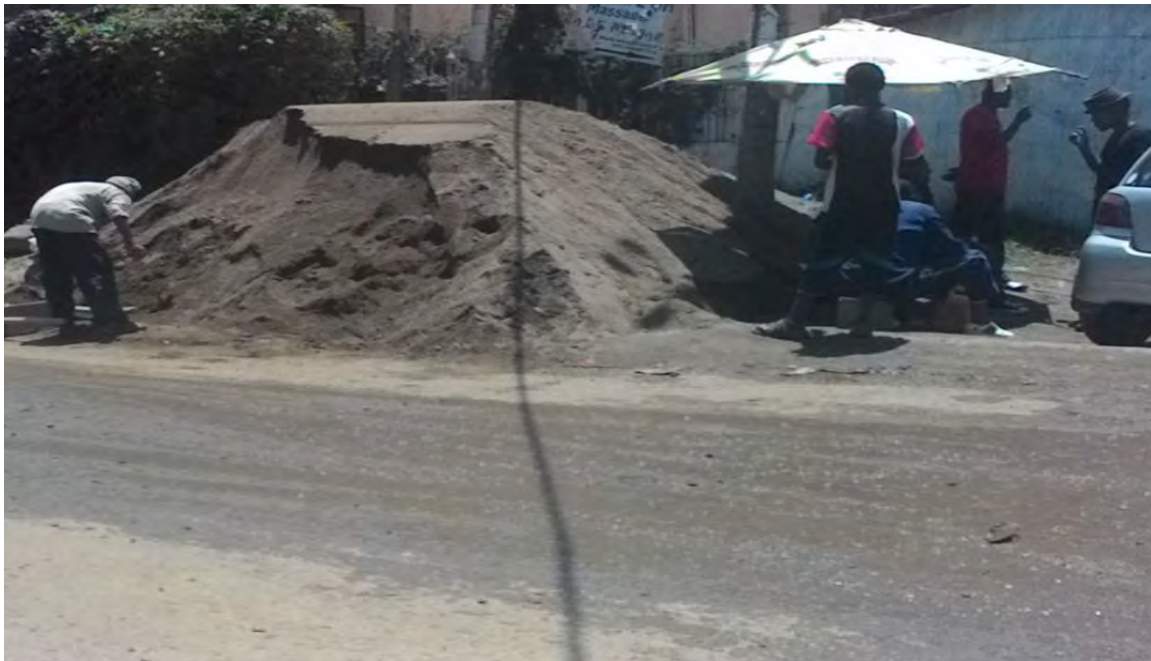
Fig.2.6 Fine Aggregates stored on side of roads
