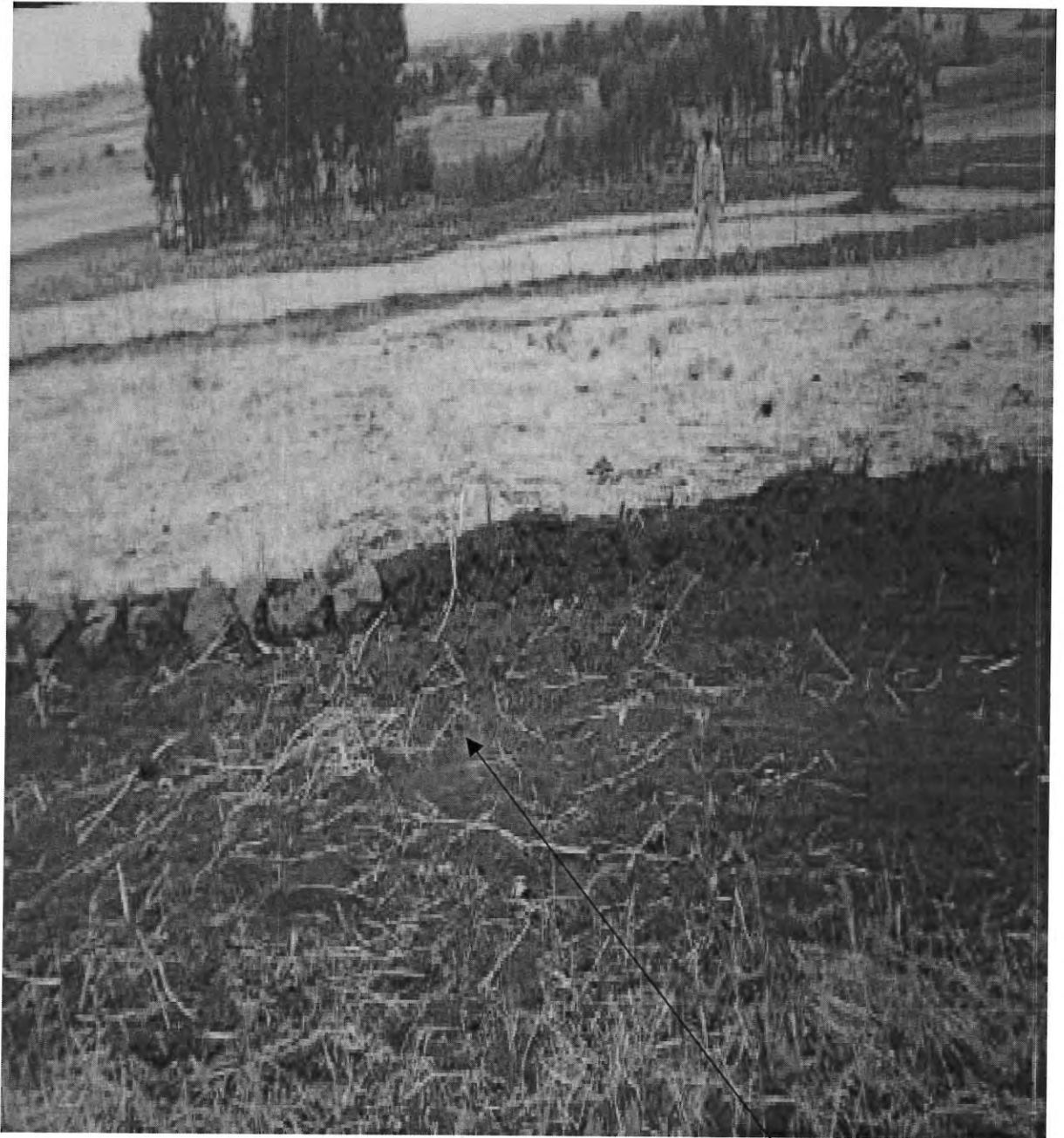
Figure -2- Bunds which were constructed but left with out maintenance and partly destroyed (Photo, taken in March, 2006)
