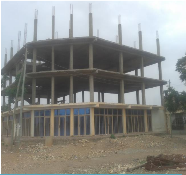
A Construction of Five star hotel
