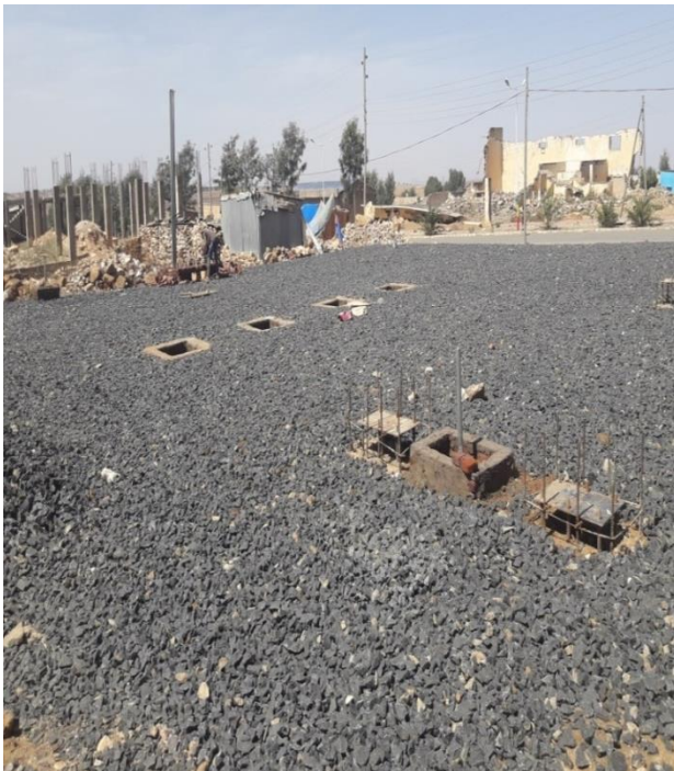
Ongoing building of oil station
