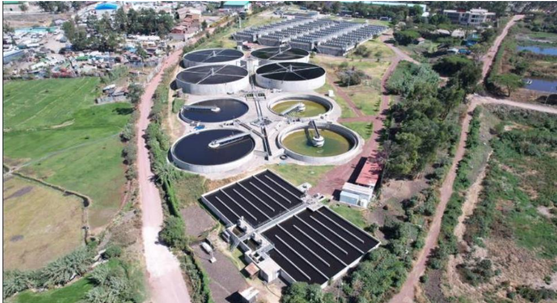
Figure 6 kality wastewater treatment plant satellite location
