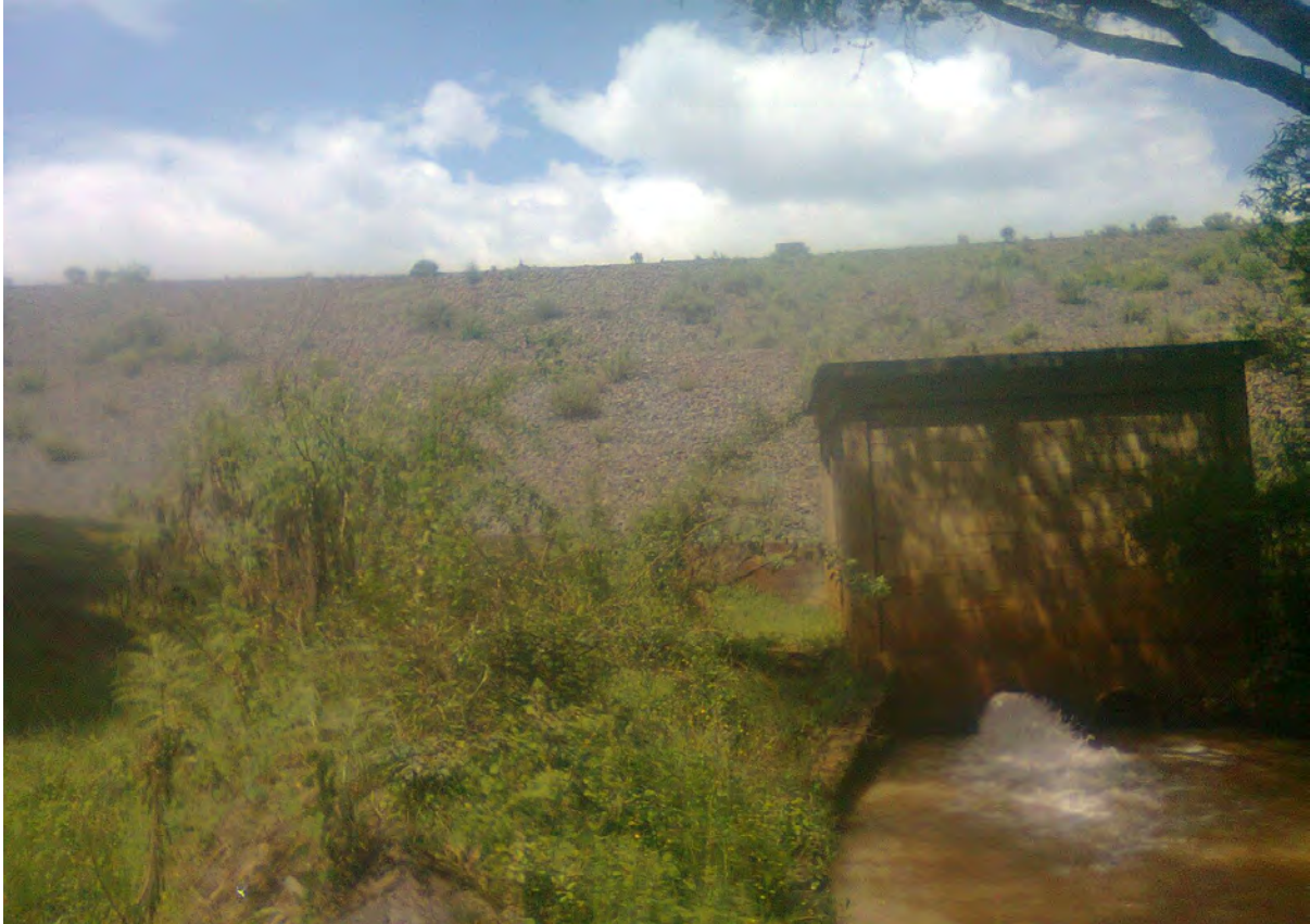
Fig 1.3 Excess water flow through the shaft spillway
