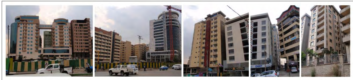
Figure 5.4: Field pictures chosen to show the very dense and congested development of the area.
