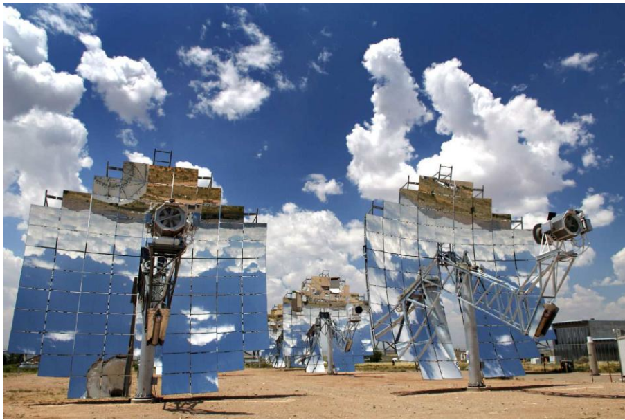
Figure 1.5 Dish Systems at Sandia National Labs (SES website, 2006)
