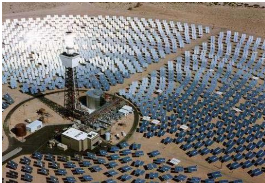
Figure 1.4 Central Receiver Systems (DOE, 2006)
