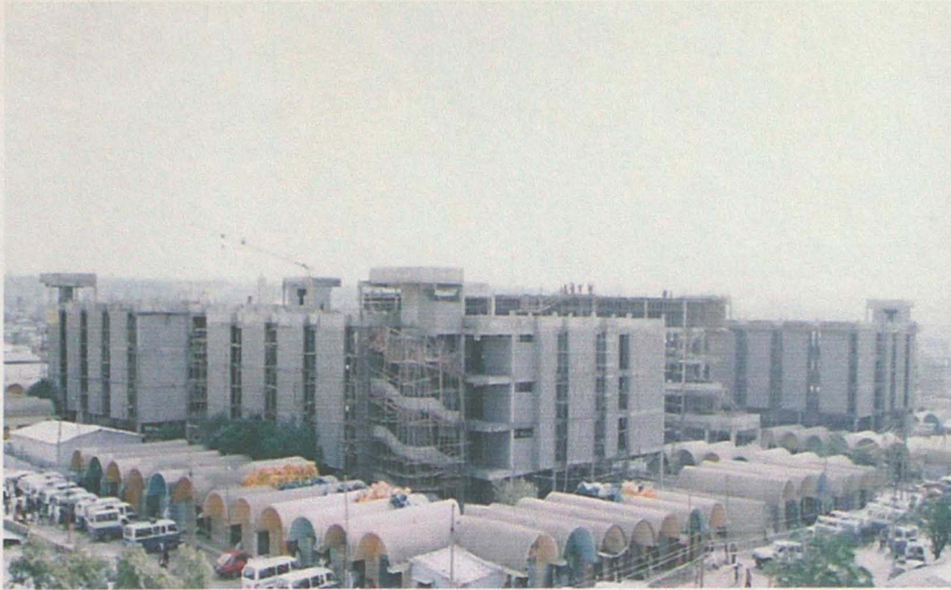
Fig.21-The Shopping complex under construction bounded by Deffeo houses
