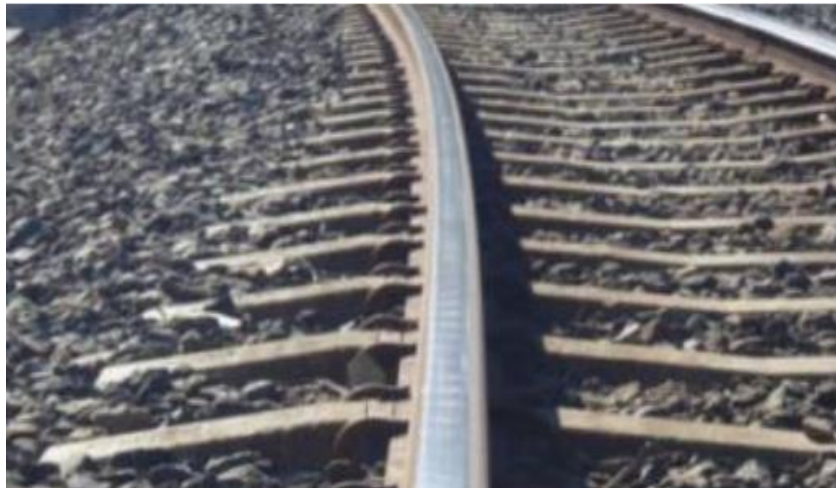
Figure 1.13. 1 – 9-month-old corrugated rail profile [22]
