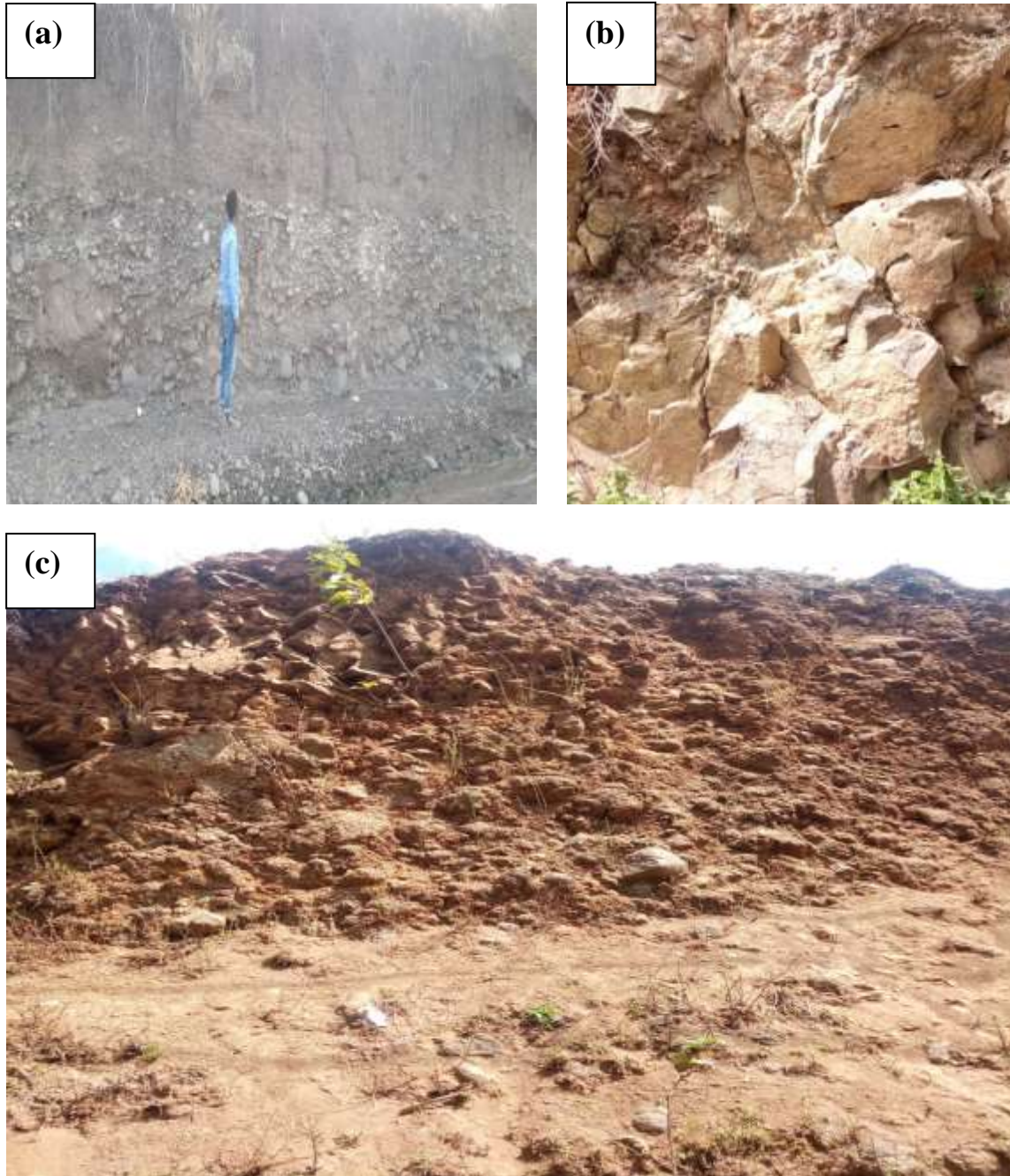
Figure 2.2: Alluvial deposit along Borkena River (a) fractured rhyolite (b) and intensely weathered basalt (c)
