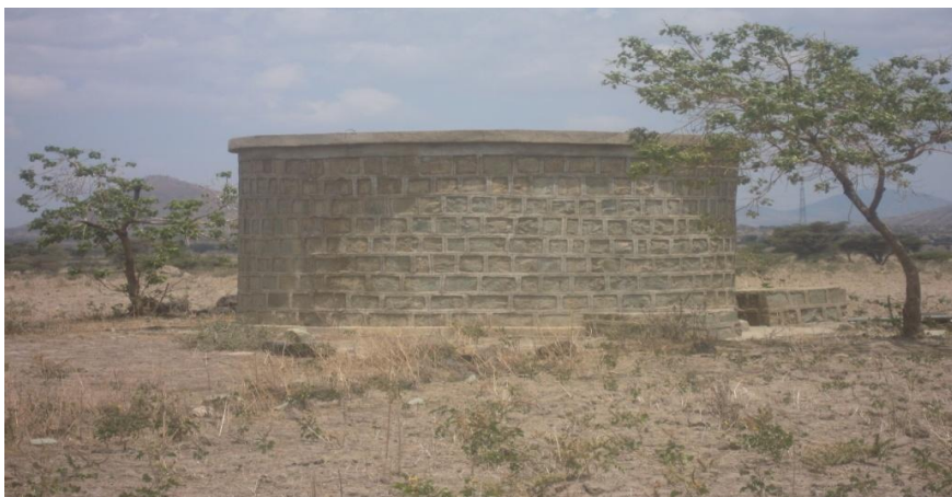
Figure 2. Reservoir constructed by ECC-SDCOM in partnership with CRS Ethiopia.
