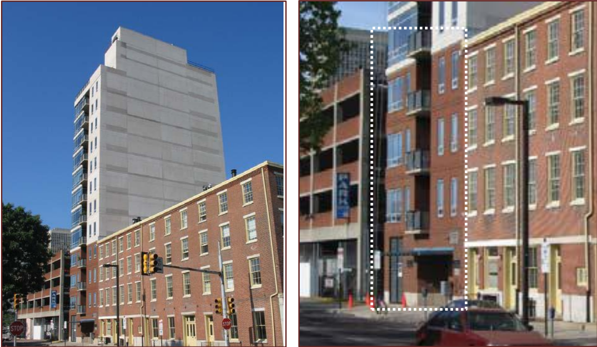
Fig. 2. 8 The Beaumont, Old City Historic District, (Preservation Alliance, 2007)
