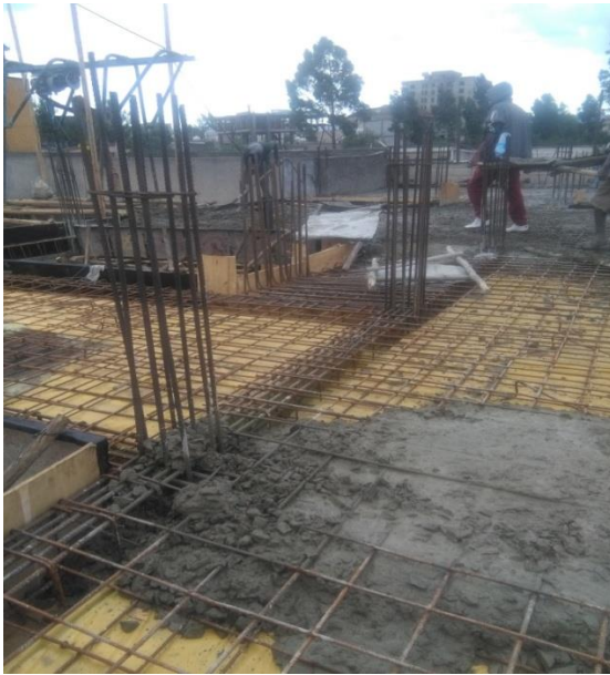
a) Building in situ cast
