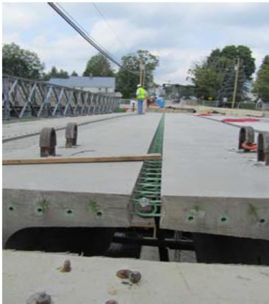
b) Bridge Connections pours with high early strength concrete
