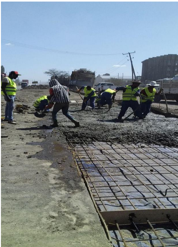
c) Road in situ cast/ rigid pavement
