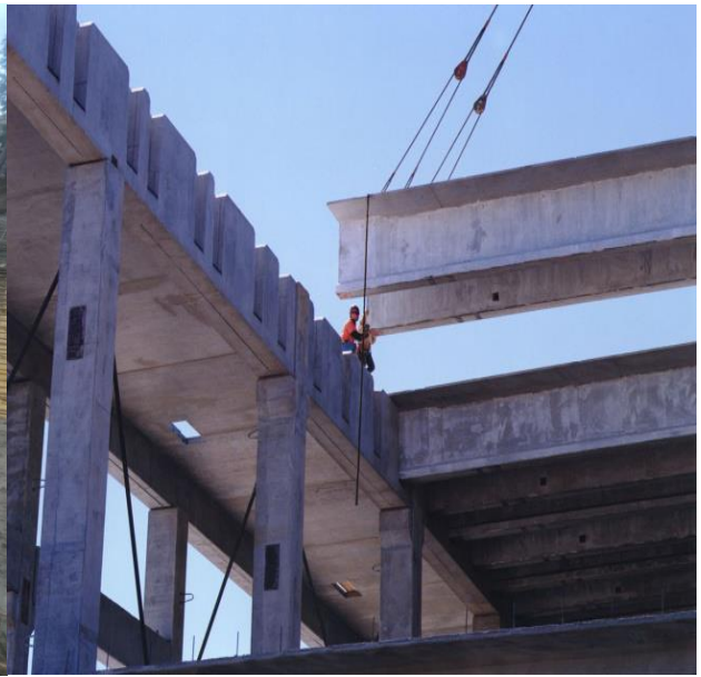
b) Building pre-cast
