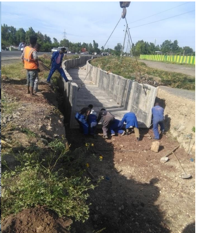
d) Road drainage Structures/ pre-cast
