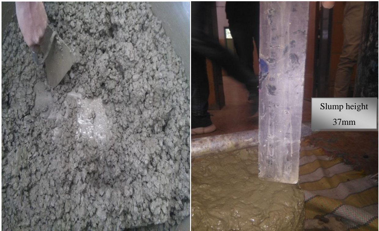
Figure 4.2: Prevailing Concrete Mix and Slump test of Conventional Concrete
