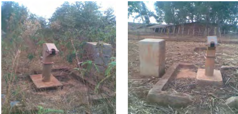
Figure 5.3 Show HDW fitted with hand pump of construction quality problem of non-functional and site selection problem in Ura kebele
