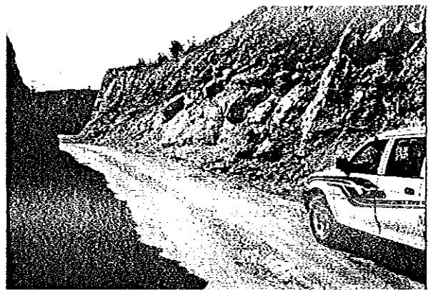
Plate 5.3 Critical soil slope section SL 10, having possible circular mode of failure
