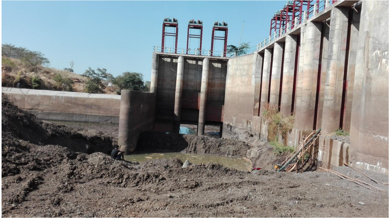
Photo 3: Under-sluice and canal head regulator of Tana Beles irrigation development project (Dec, 2017)
