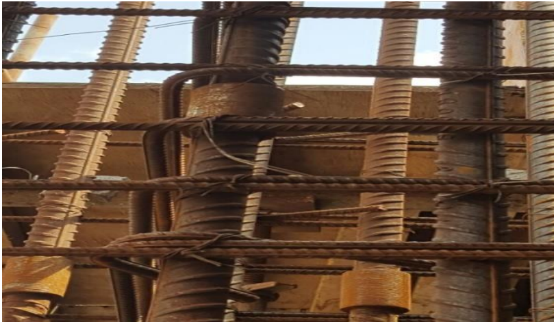
Figure 4.3: Mechanical Splice Reinforcement Steel (photo Adey Abeba Stadium from Geriji Emprial)
