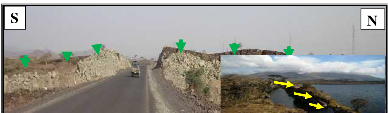
Plate.2.7. Topographic feature and extended fissure and fractured zone
