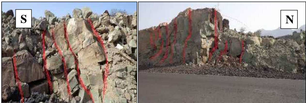
Plate2.5.Fissures and fractured zones running in a N–S direction crossed by the new road.
