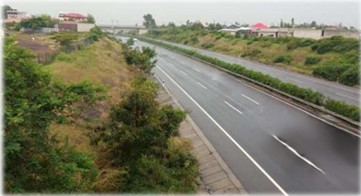
Figure 4.22: Addis Adama Expressway Passing through the town
