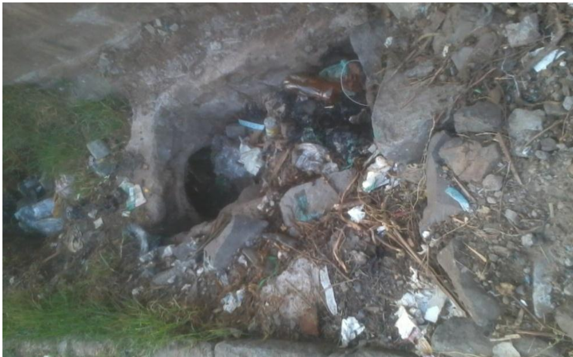
Figure.1.1. Drain blocked by solid waste, Wereda nine saint Rufael church area (photo: Researcher's field observation, 2014)
