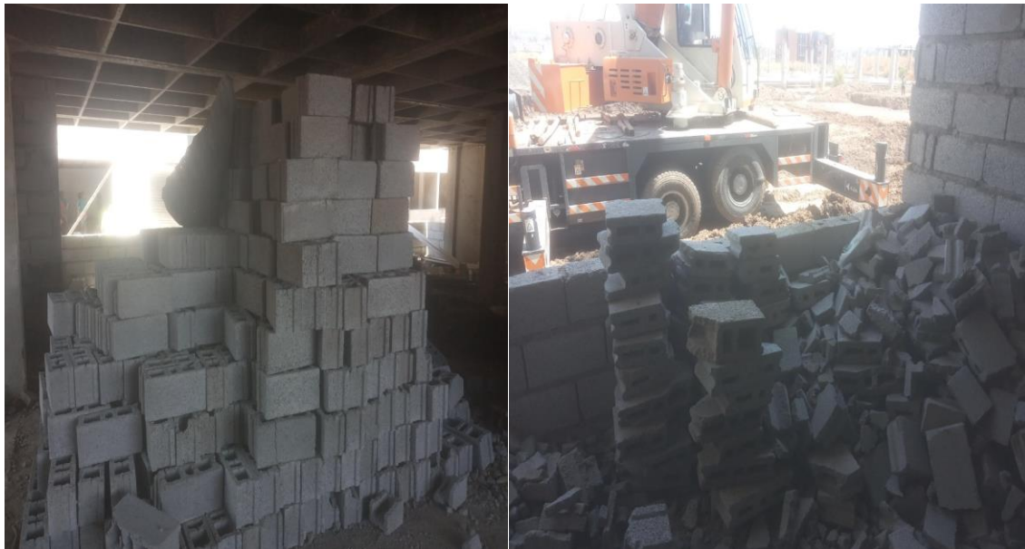
Figure 4-5: Inappropriate storing of HCB
