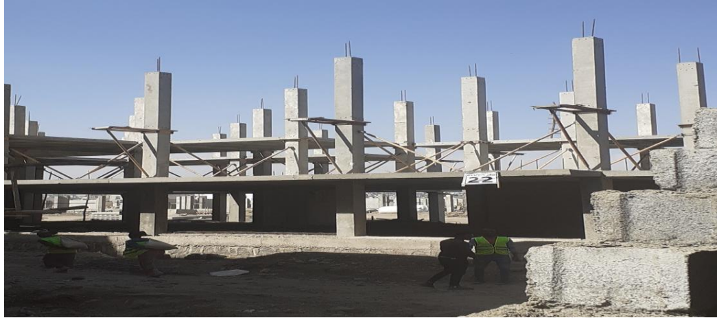
Figure 4-6: Not timber formwork used in prefabricated site
