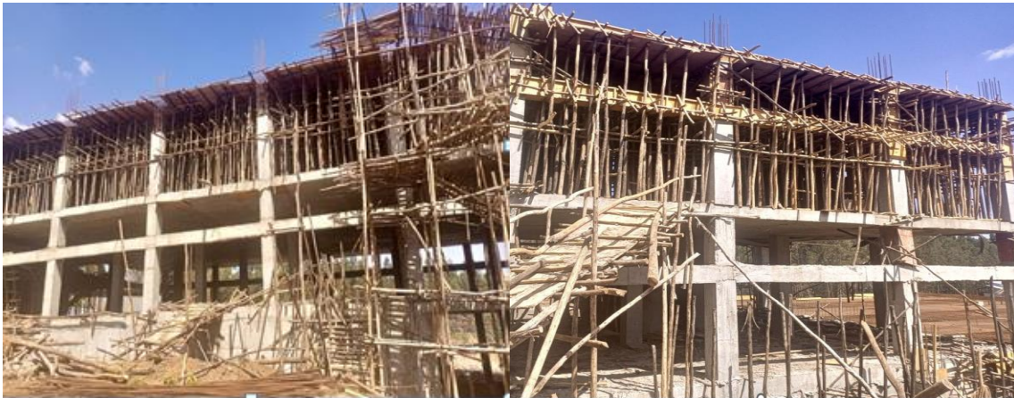
Figure 4-7: High amount of timber formwork used in on-site construction site
