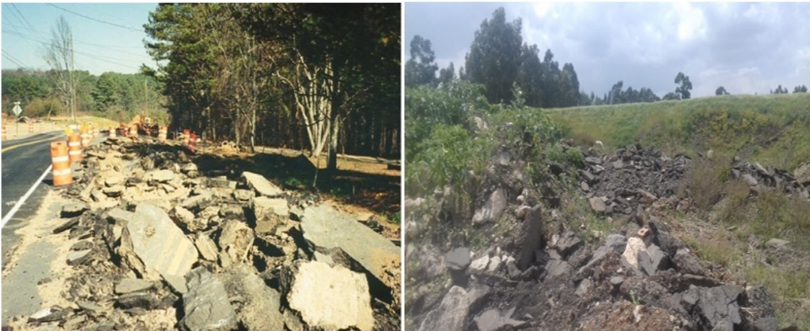
Figure 2.4: Pavement rubble from full depth demolition of roadway
