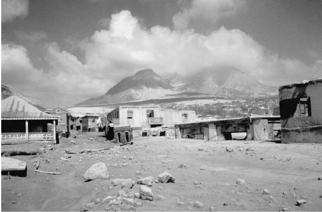
Figure 3.2 Looking eastward from the site of the former capital city of Plymouth, near Sagar Bay on the southwestern side of Montserrat. Structures have been damaged and destroyed by a combination of pyroclastic flows and lahars. Soufrière Hills Volcano is visible in the background; the pyroclastic flows originated from collapse of the unstable lava some located between the two prominent peaks. (Photograph by Richard P. Hoblitt, US Geological Survey).
