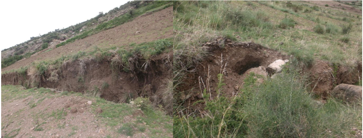
Figure 15: Gully caused by land degradation within the study area
