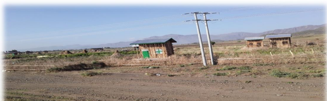
Figure 4 Illegal building on farm land
