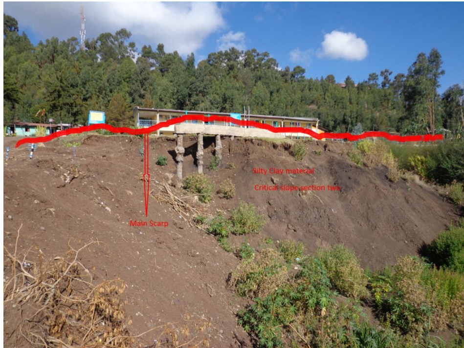
Plate 4.2 Sliding of silty clay soil along Critical slope section SS2
