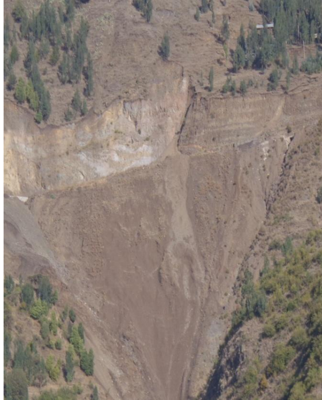
Plate 3.5 Removed toe support for Road construction
