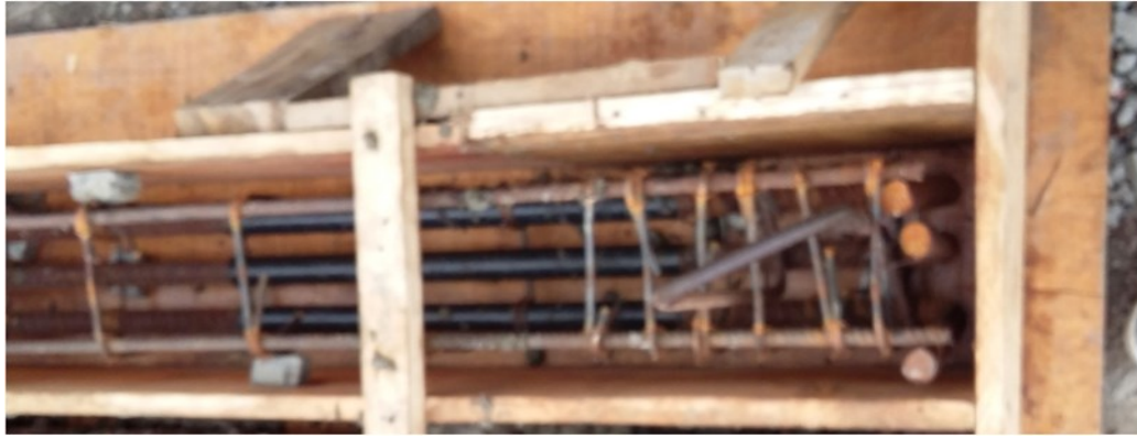
Figure 3-13: Reinforcement cages inside the formwork
