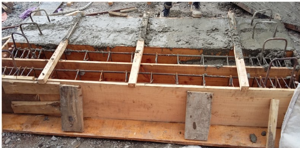
Figure 3-14: Concrete placing process
