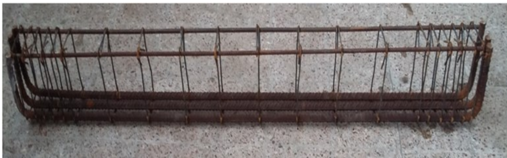
Figure 3-9: Reinforcement cage of full span bonded beam
