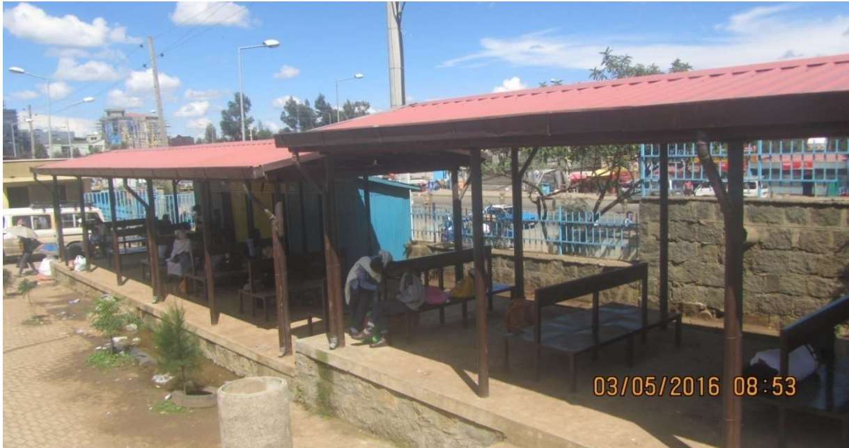
Figure 4.4 Passenger waiting area at Lamberet Terminal
