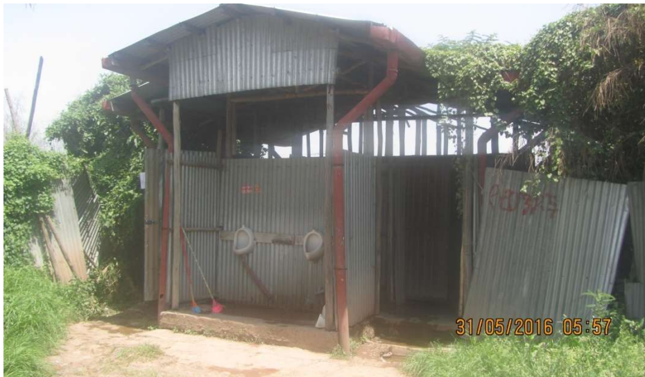
Figure 4.3: Passenger restroom at Kality Terminal
