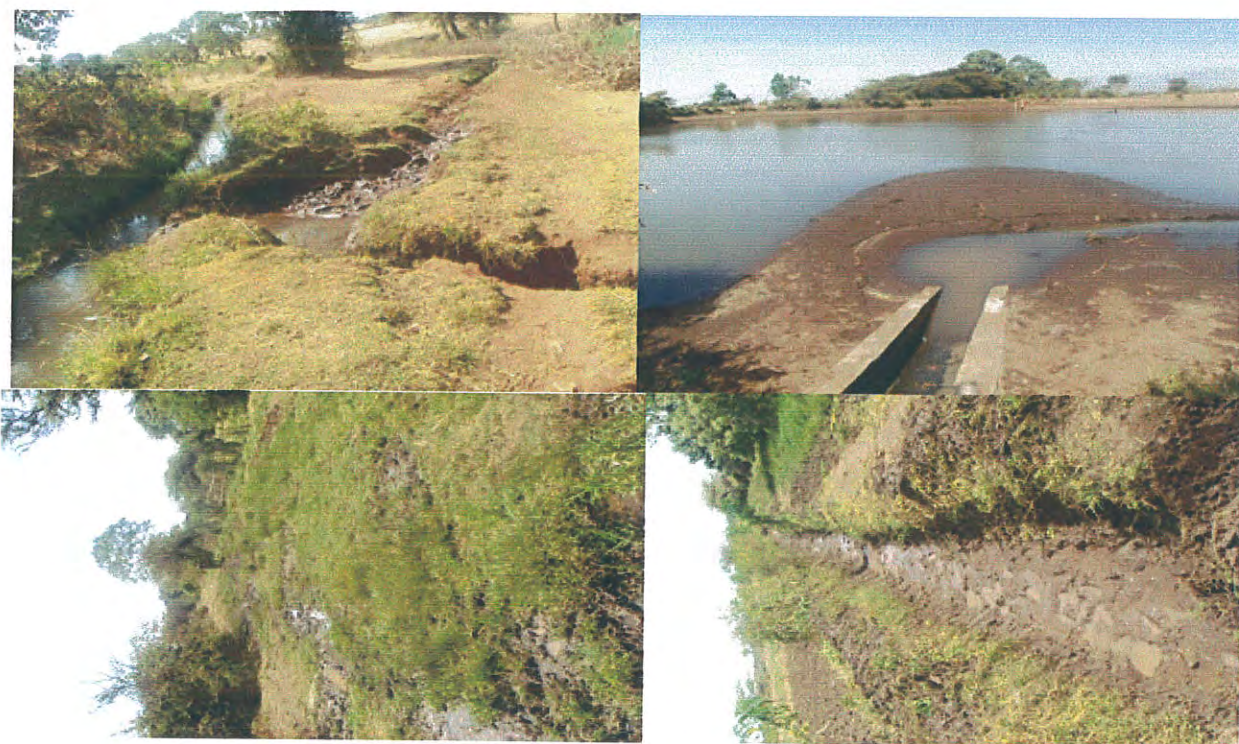
Figure 18 Effects of Canal structure Problems on Water Resource Managemen
