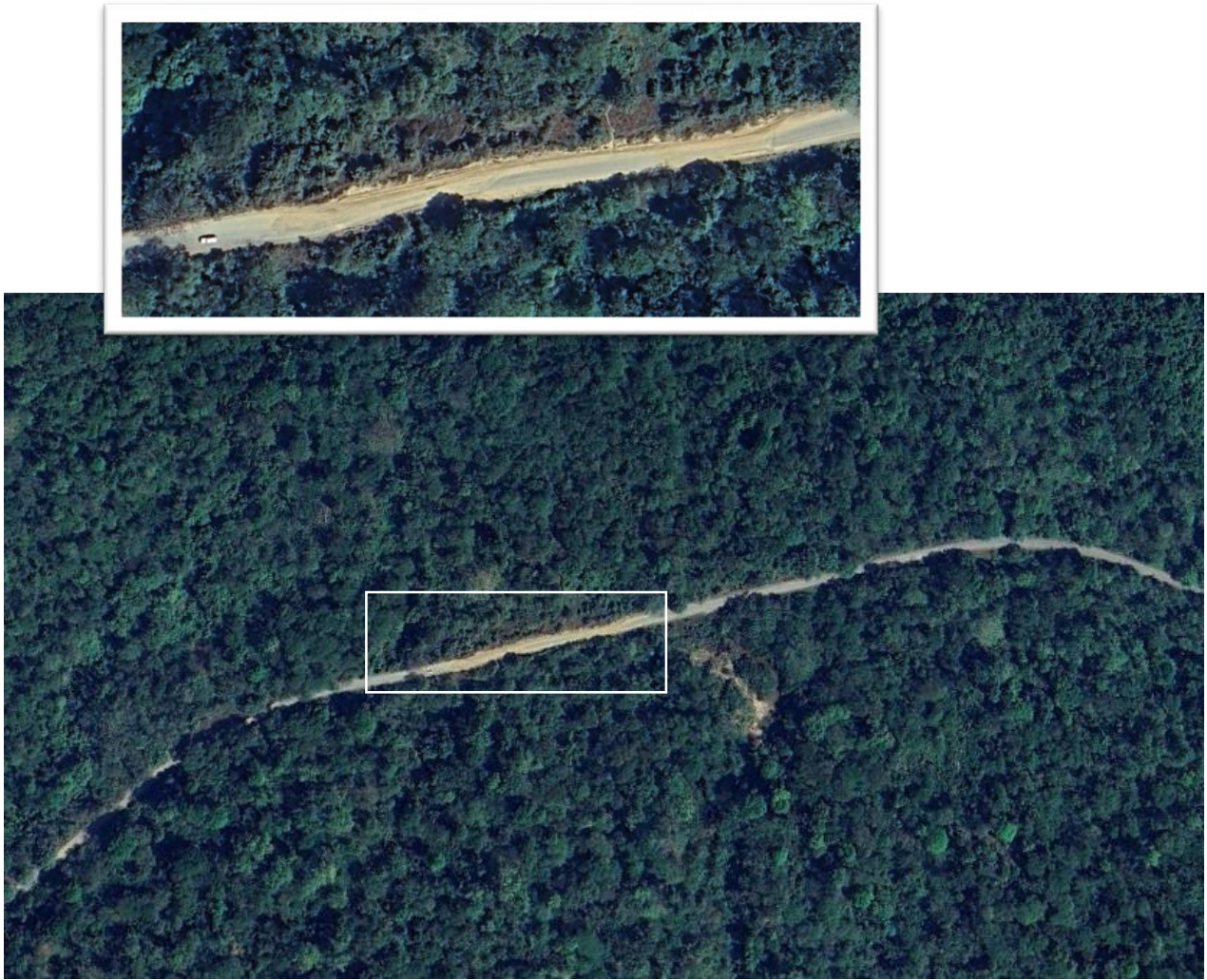
Figure 4-16: Landslide affected road section at 48+800 [Source – Satellite Image by Google Earth]
