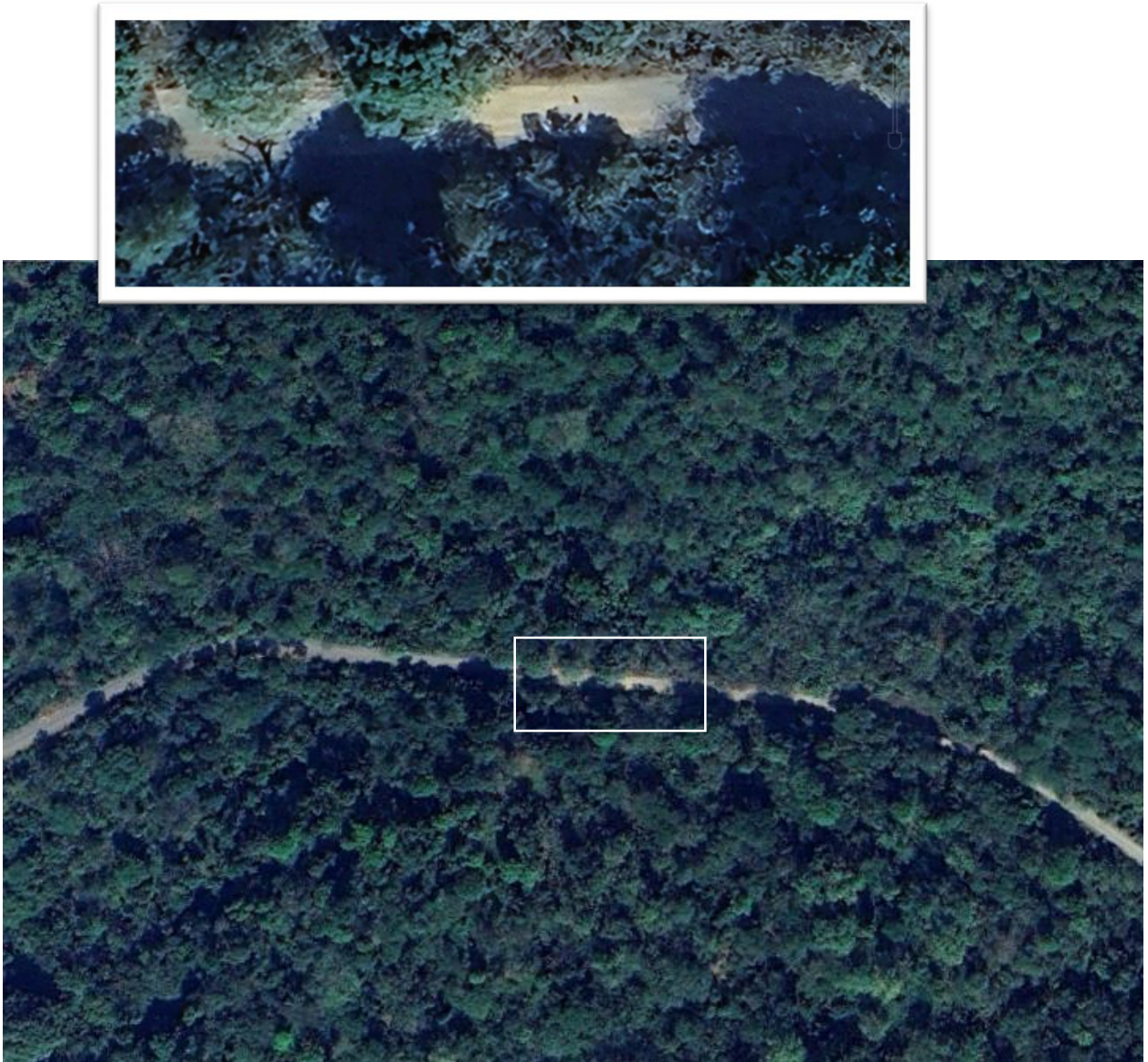
Figure 4-18: Landslide affected road section at 49+000 (Achebo/Dawe) [Source – Satellite Image by Google Earth]
