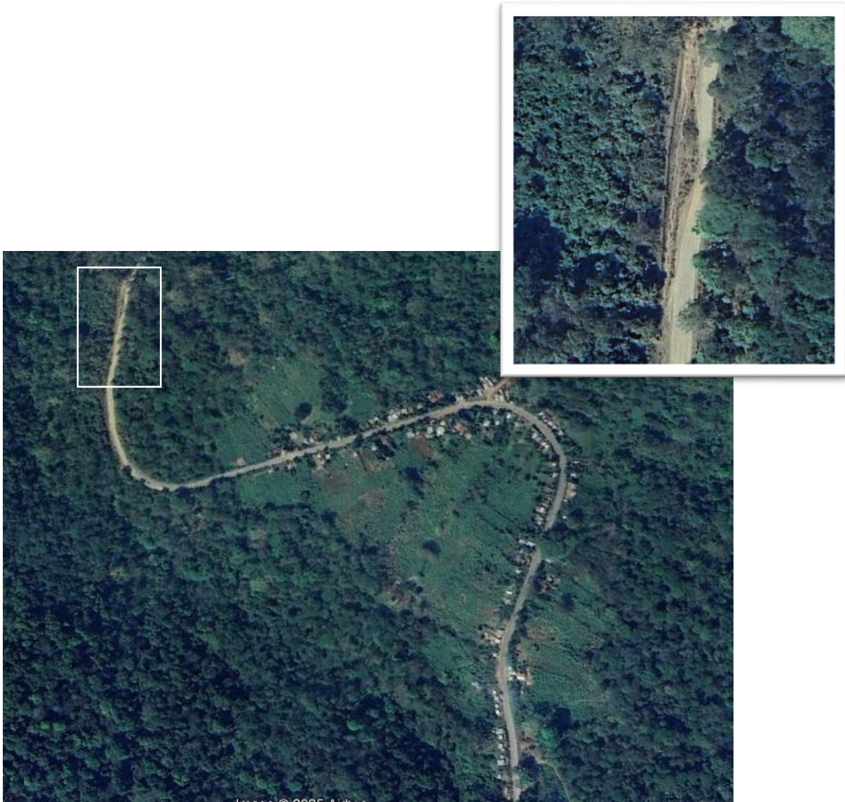
Figure 4-9: Landslide affected road section at 44+000 (inside "Yayo Forest") [Source – Satellite Image by Google Earth]
