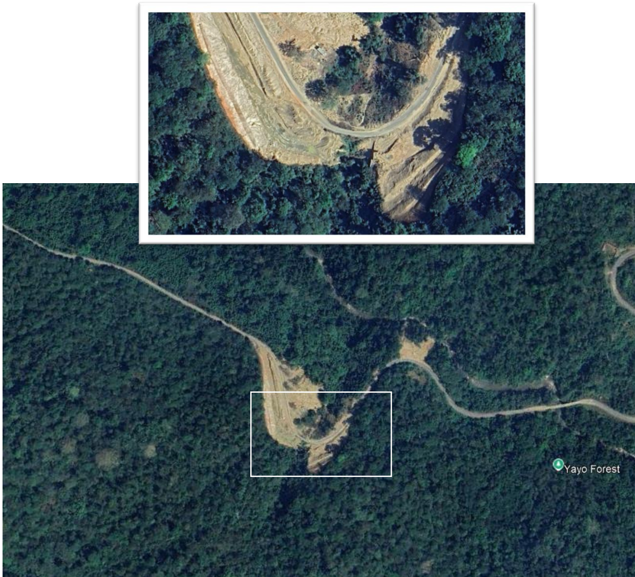
Figure 4-14: Landslide affected road section at 46+920 (Yembo) [Source – Satellite Image by Google Earth]
