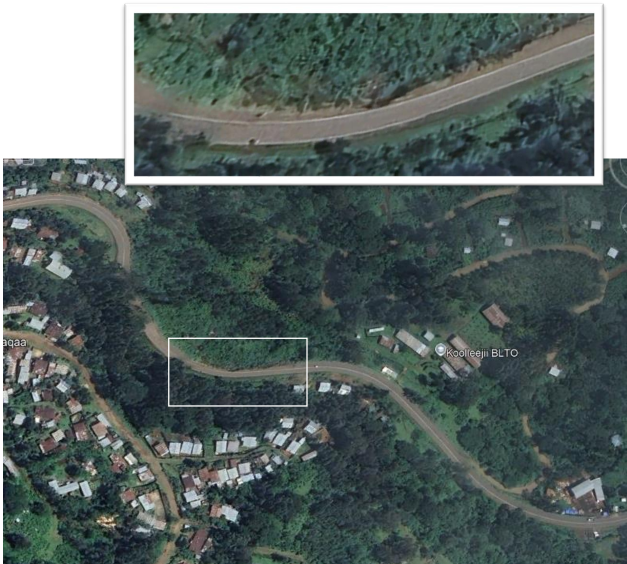
Figure 4-26: Landslide affected road section at 201+700 (Gore) [Source – Satellite Image by Google Earth]
