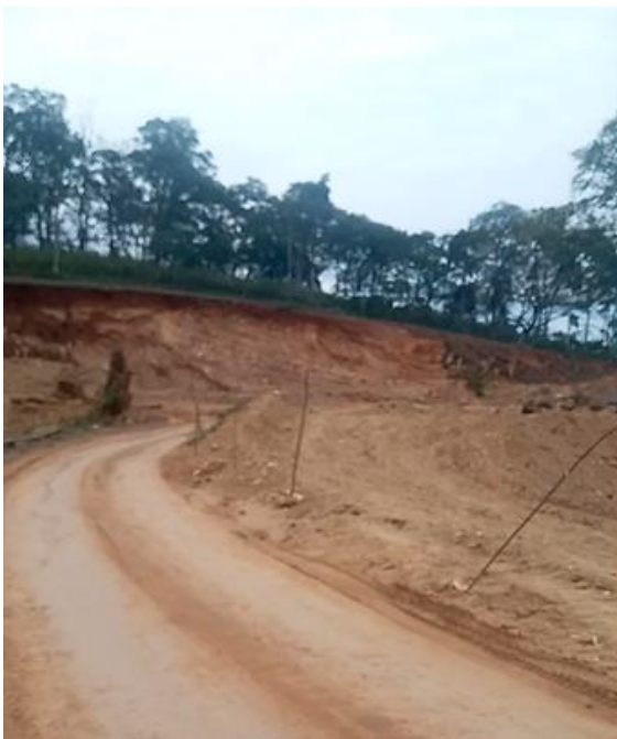
a) Large volume of selected fill material application downstream of the roadway
