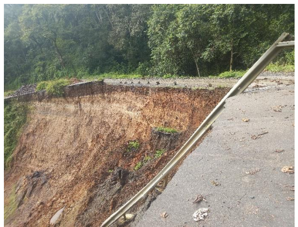
Figure 4-12: Land slide at 46+920 (Yembo) before any remedial measure taken [Source – historical pictures of onsite investigation by ERA engineers]
