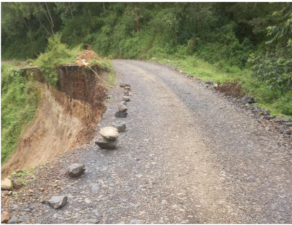
Figure 4-12: Land slide at 46+920 (Yembo) before any remedial measure taken [Source – historical pictures of onsite investigation by ERA engineers]
