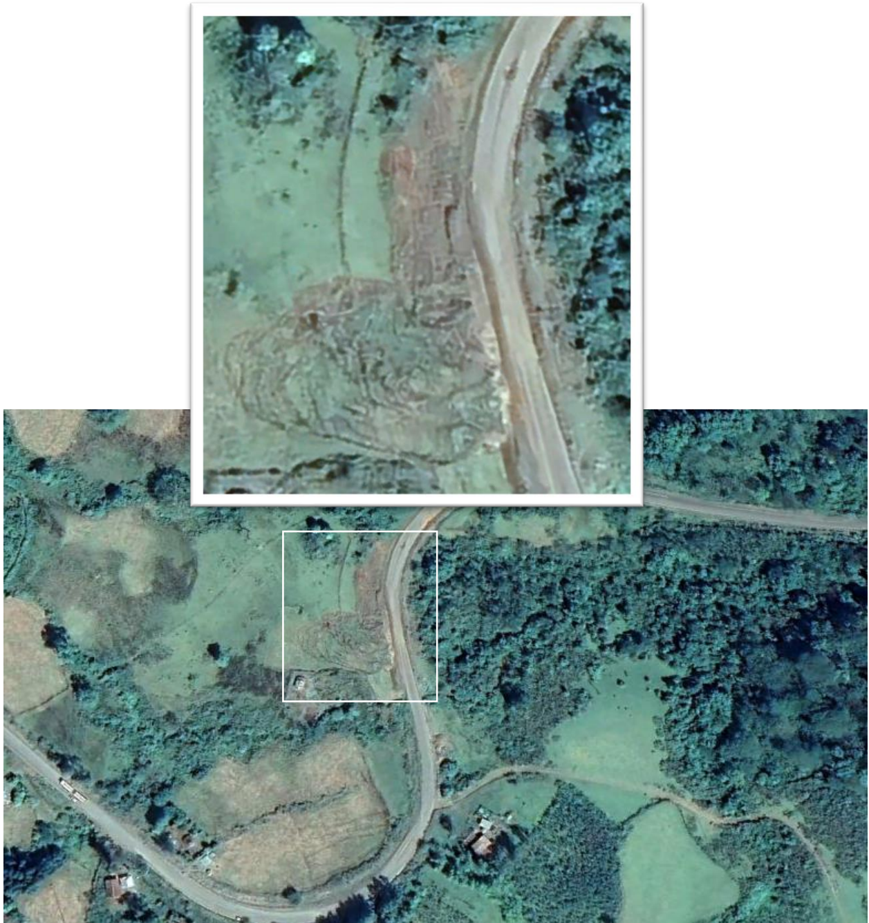
Figure 4-24: Landslide affected road section at 85+550 Hurumu/Gaba [Source – Satellite Image by Google Earth]
