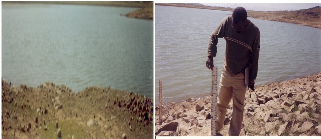
Figure 4.1 Photographs Showing the Different Views of Haiba Reservoir
