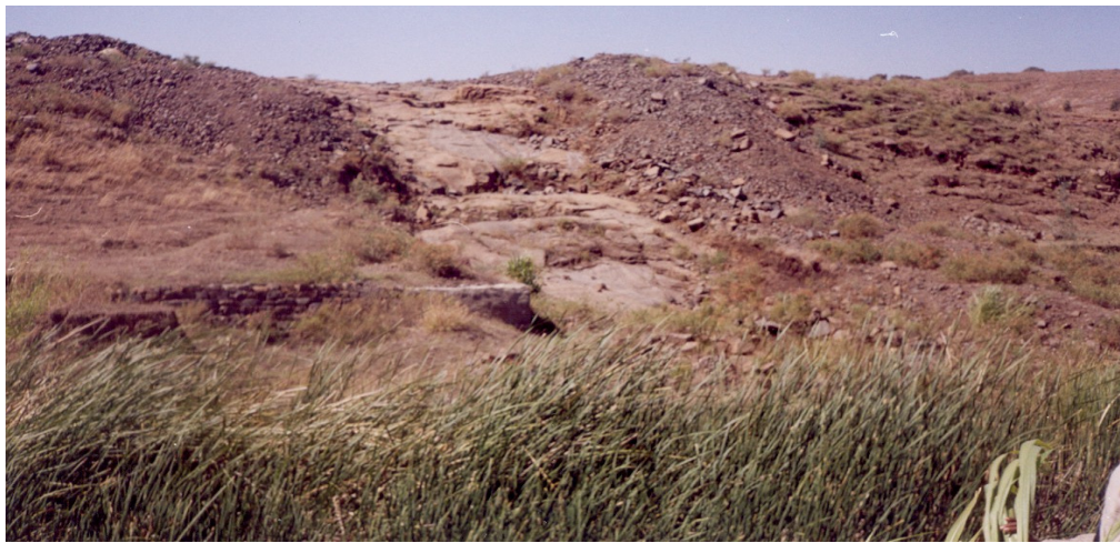
Figure 4.3 Photograph Showing Part of Spillway
