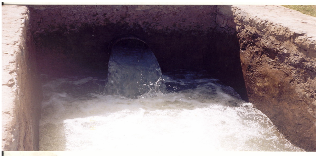
Figure 4.4 Photograph Showing the Irrigation Outlet
