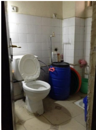
Figure 2.19 Way of toilets arrangement in most condominiums of Addis Ababa
