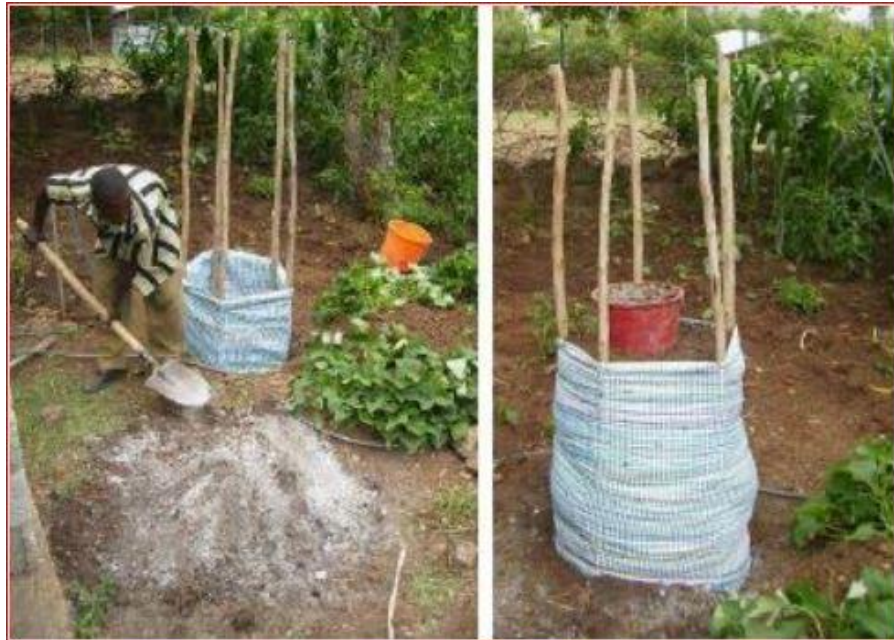
Figure 2.3 (Right) Preparation of greywater tower in three steps: mixing soil, ash and compost, (Left) filling the gap(ROSA, 2010).
