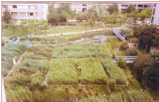
Figure 2.9 Constructed wetland used to treat greywater from a housing development in Berlin, Germany (Nolde 2005)
