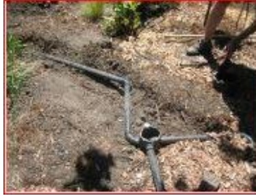
Figure 2.15 Branched drain system (Allen, 2018).
