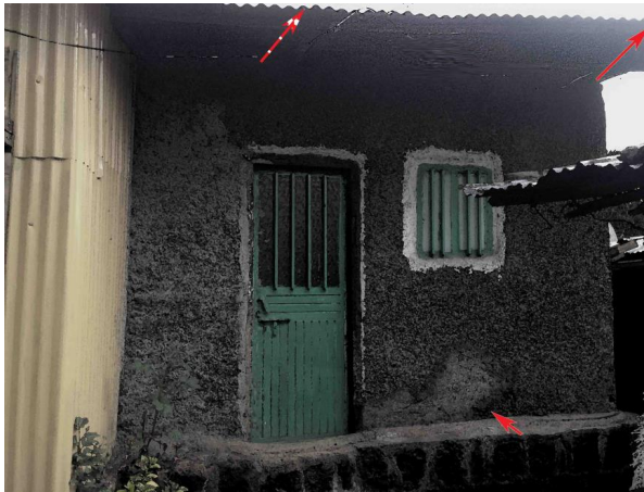
Figure 5 Common Type of Kebele Housing with Attached Unit with CIS Wall and the Narrow Paths of the Neighborhood
