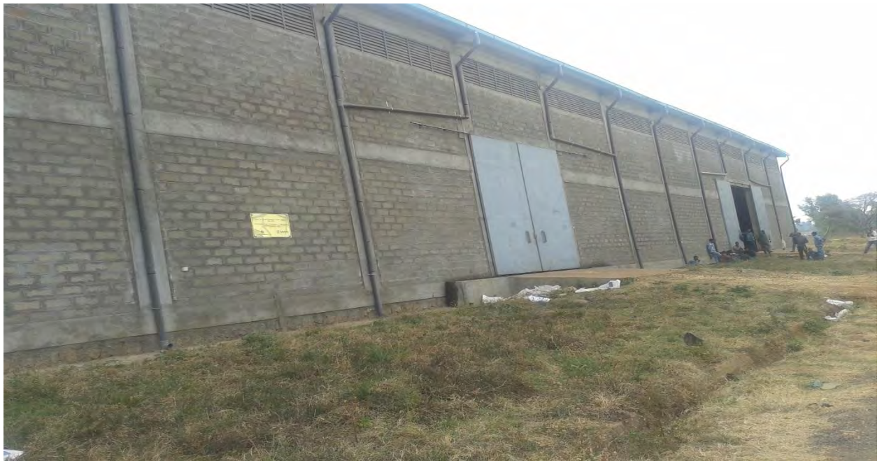
Photo 10. Gibe Dedessa grain warehouse
