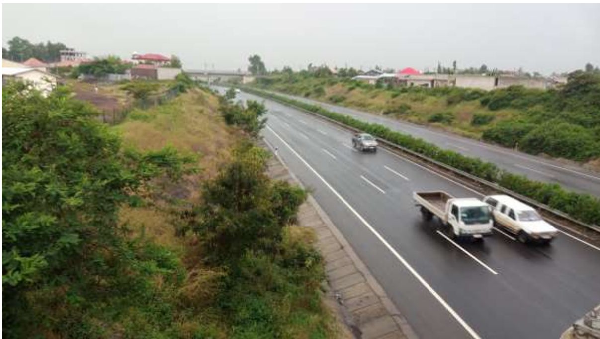
Figure 4.28: Showing Addis-Adama expressway passing through the town (Source: Own photo, 2020)
