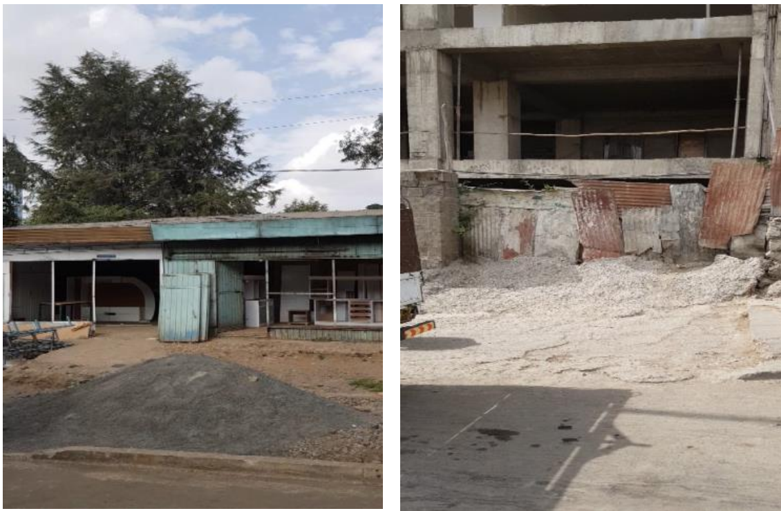
Figure 4. 22: Image showing construction site debris obstructing the pedestrian ways
