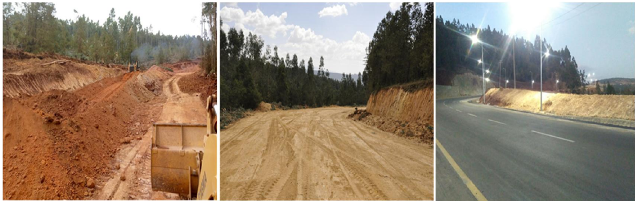
Figure 19: Kuskuaam – Entoto Road Project Progress
