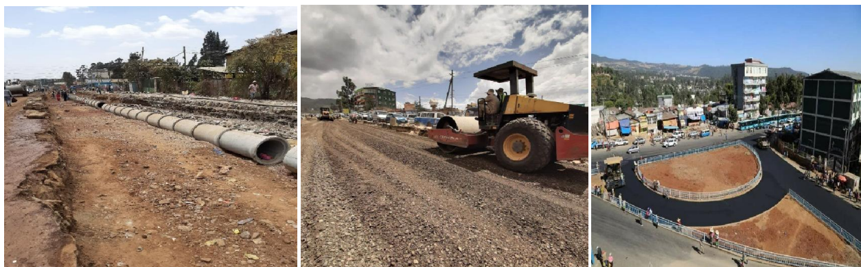
Figure 20: Shiromeda - Kuskuam Road Project Progress
