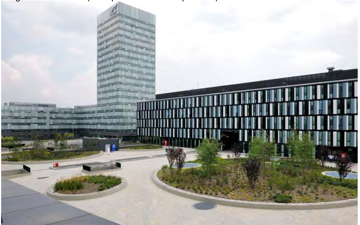
Figure 4.4: Exterior facade view of B-5 building
