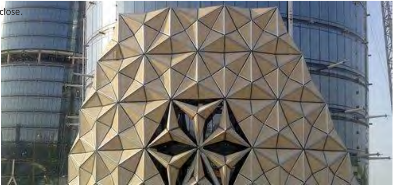
Figure 4.2: Automated Opening and Closing illustration of shading system – real photo
