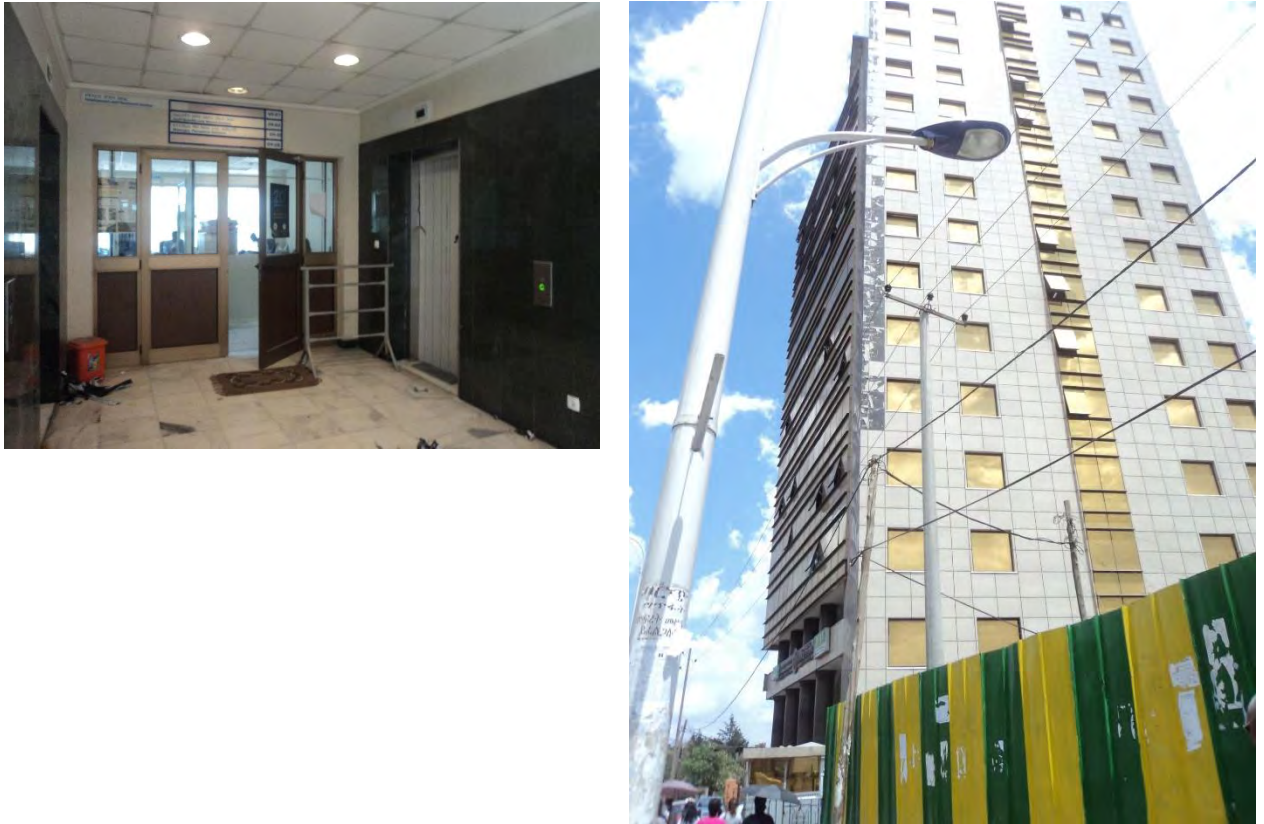
Figure 3.7: Interior and Exterior feature of Debrework Tower
