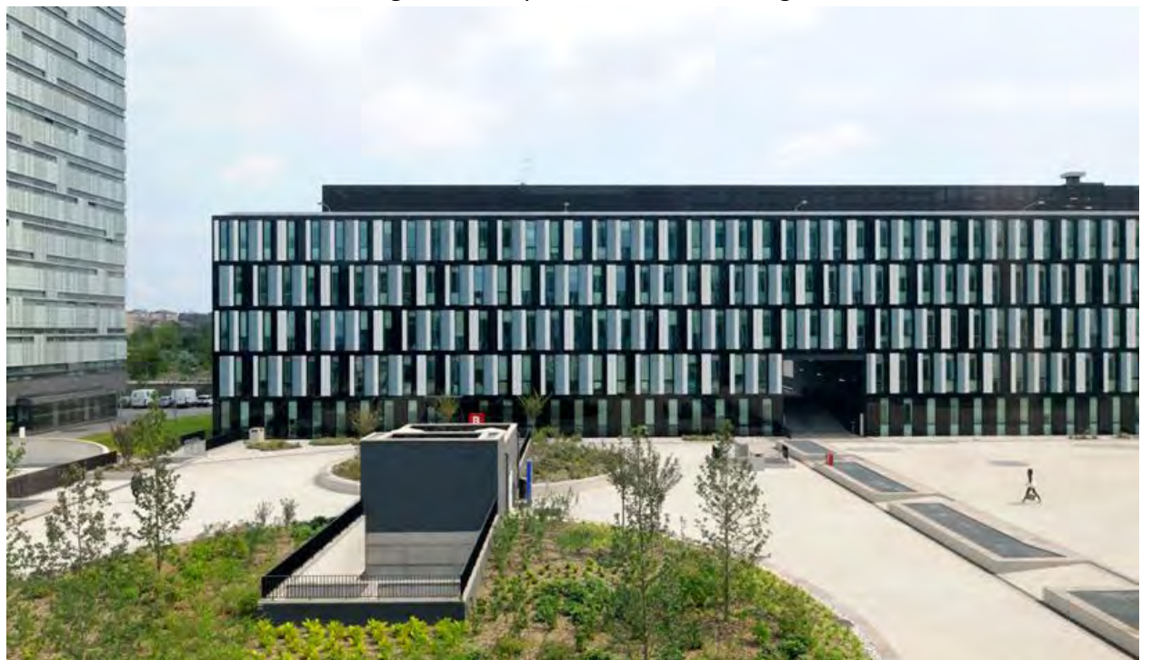
Figure 4.7: Exterior facade view of B-5 building
