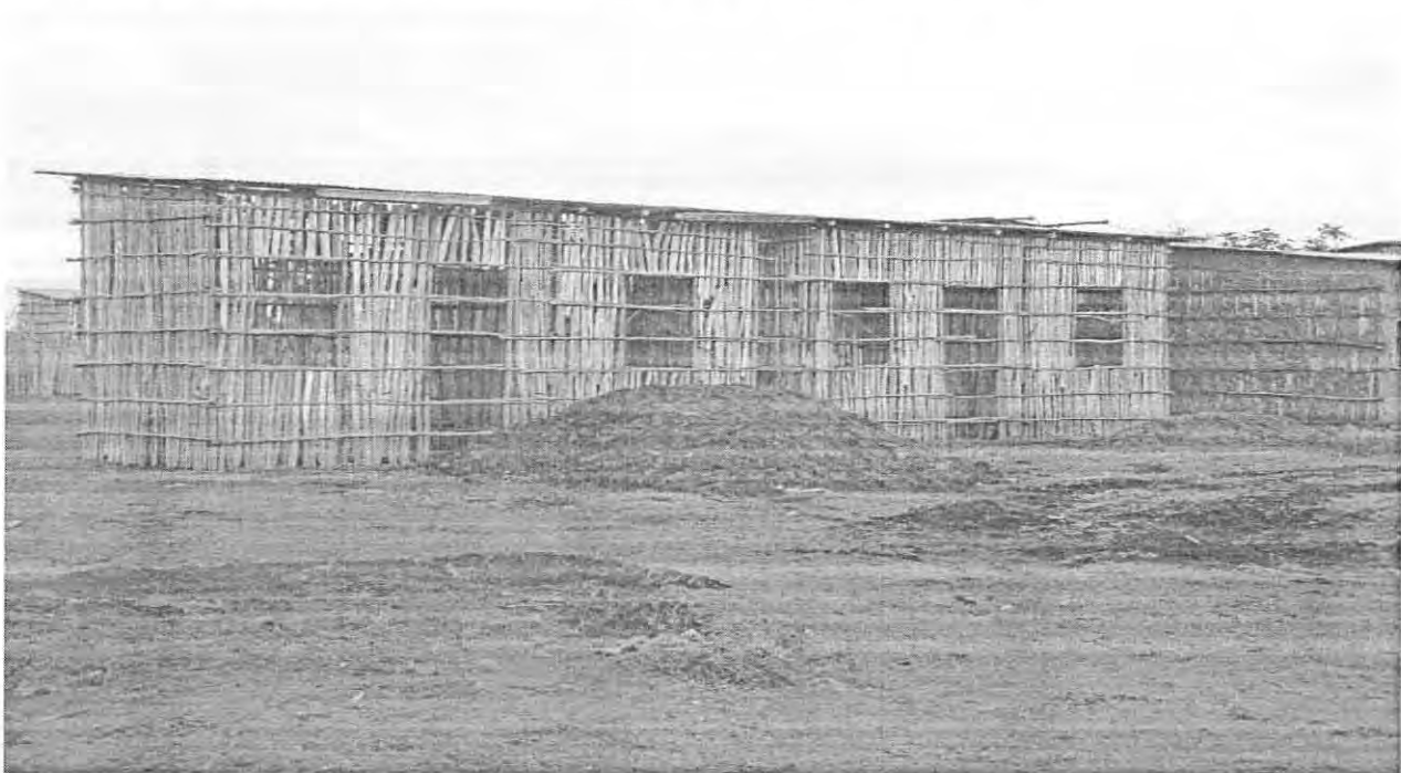
Picture 5.3 a house under construction in Dato kebele during field survey
