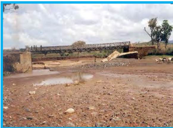
Photo 11: Delbena River Bridge (Aug 2006)
