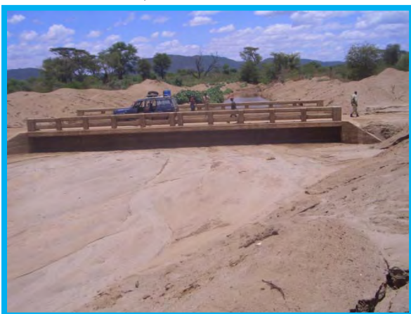
Photo 16: Aggradation on river Segen with inadequate opening (Aug 2007)
