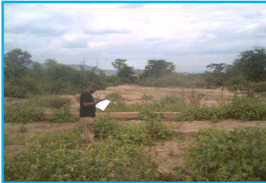
Photo 5: Segen River Bridge completely buried under sediment (Aug 2007)
