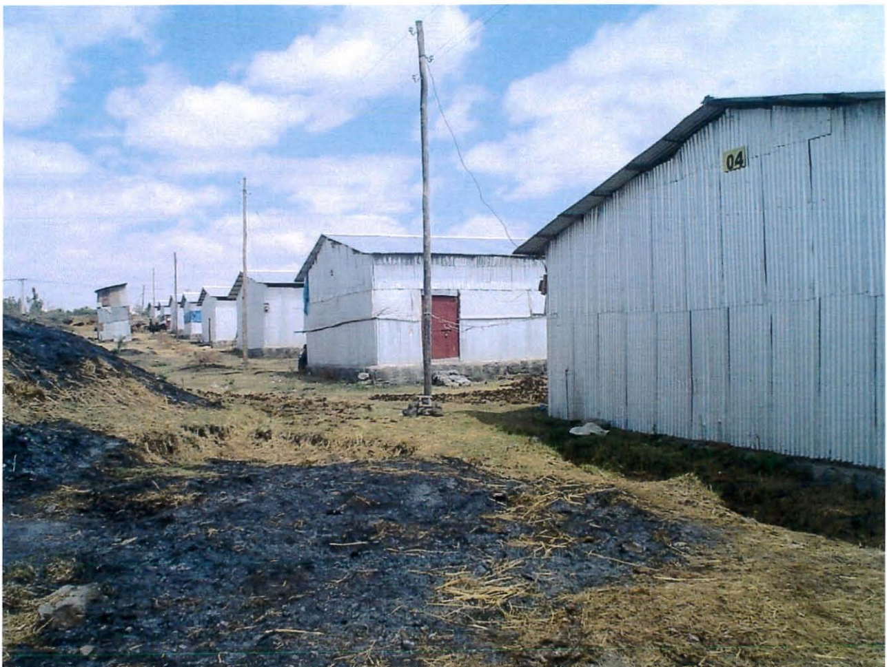
Figure 7: Outside view of the shades constructed by Woreda 01
