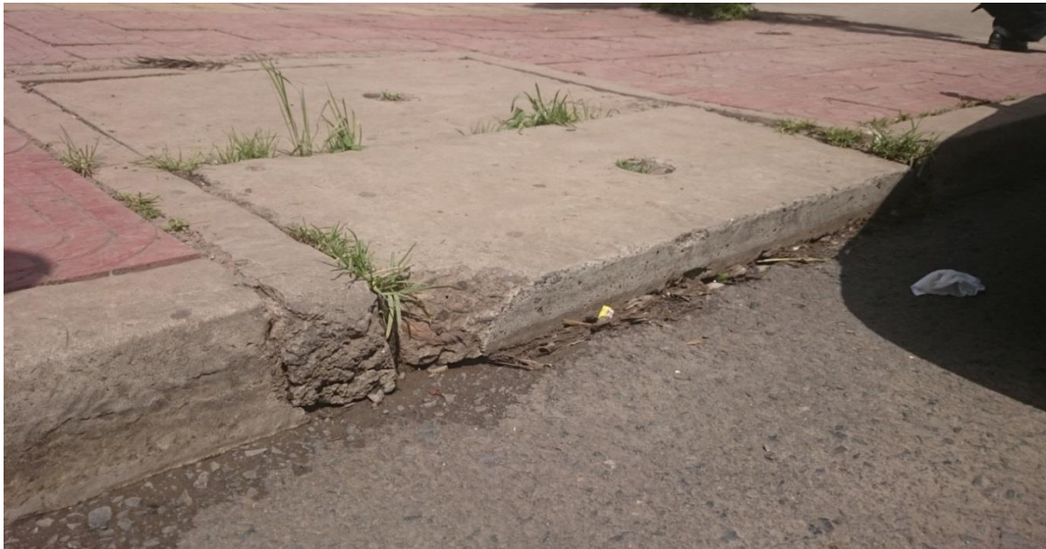
B. Manhole opening closed with muds/Garbage
