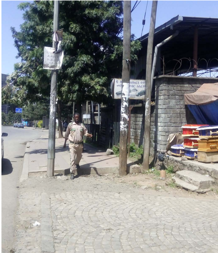
Figure4.Example of inaccessible pedestrians' pavement with unnecessary electric poles around the the way along theentrance of ENADB.
