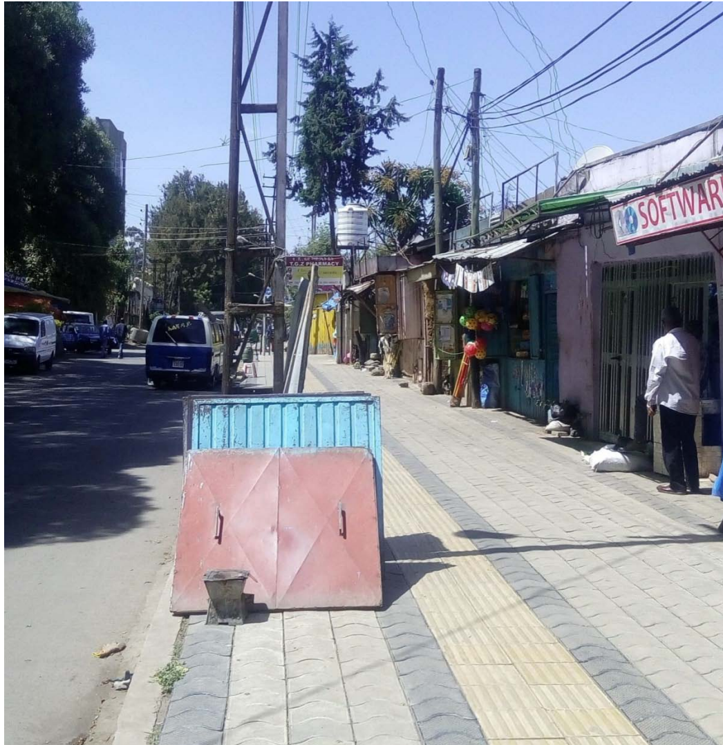
Figure 8. Example of inaccessible electric pole at pedestrians' pavement around the ENADB.
