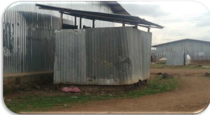
Plate 4.2: Private Household's kitchen and toilet constructed beside the main housing unit
