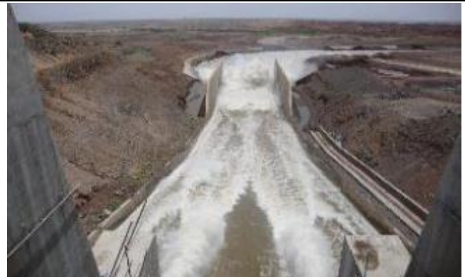
4: Flow along the chute
