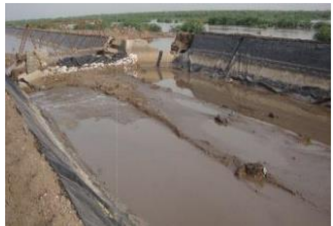
2: Canal Breach at Main Canal (MC)
