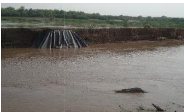
5: Canal Breach at Main Canal (MC)
