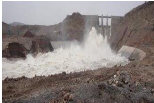
6: Flow after Stilling Basin
