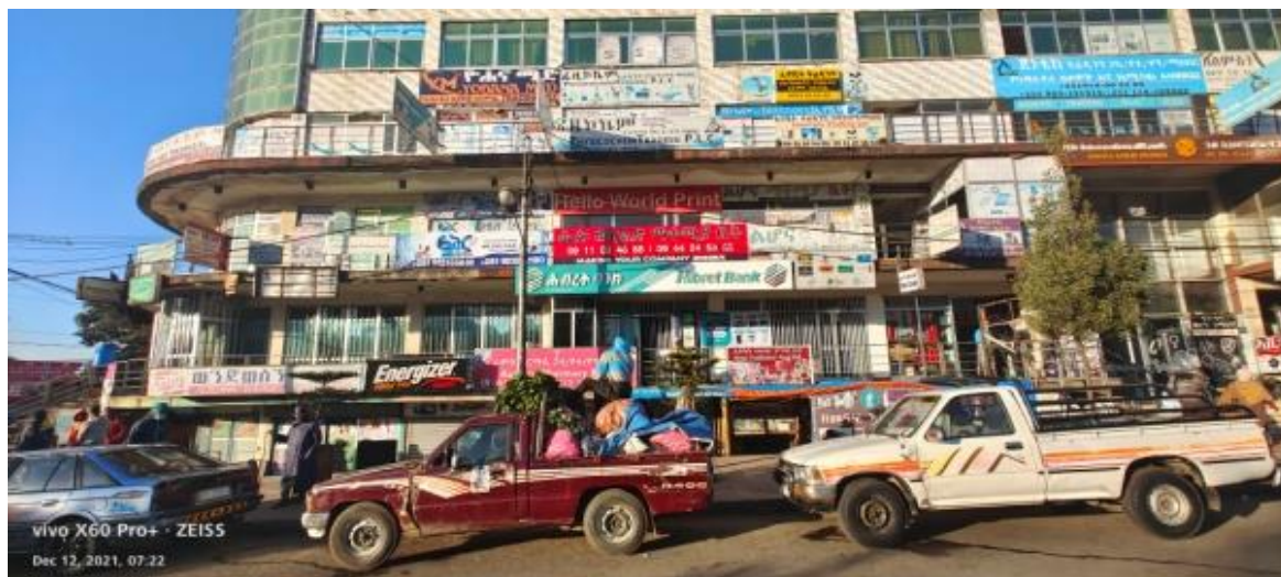
Figure 6.7: Photo showing signage on a building (Lemat le edget) at Sebara babure
