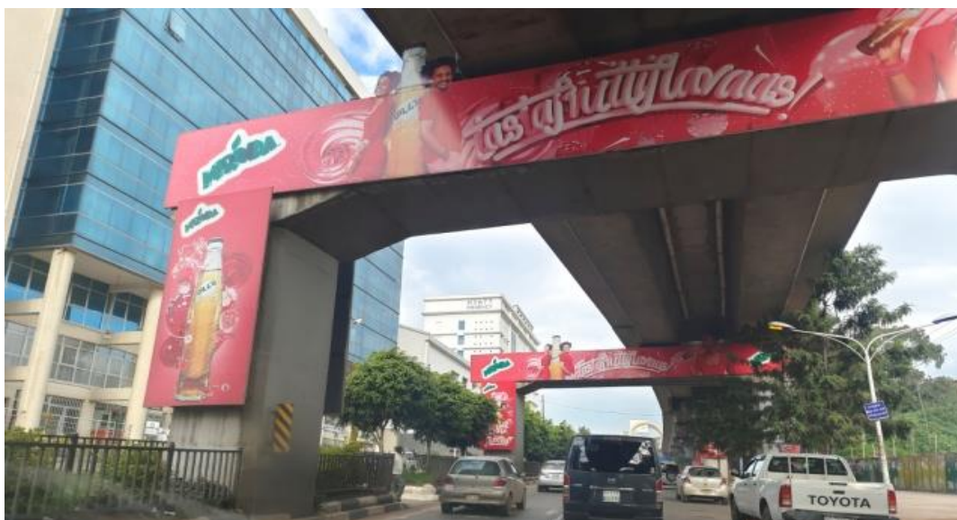
Figure 6.6: Photo showing signage on the structure of the railway in front of Mariot Hotel
