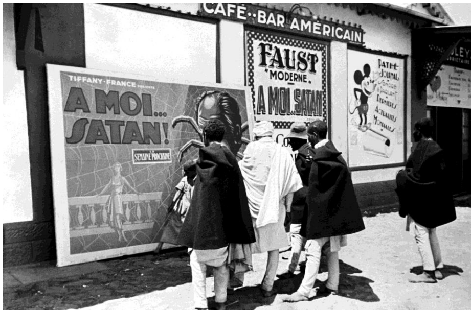
Figure 6.2: Outdoor Signage in early Addis Ababa
