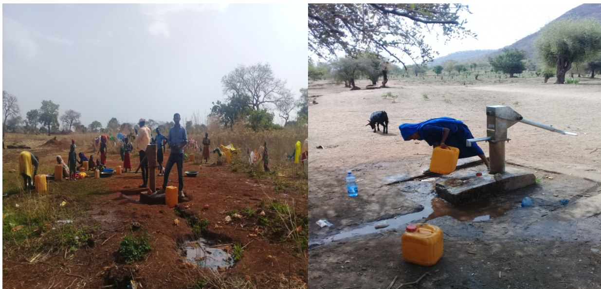
Figure 6: Hand pump without fence in both water points and top work crack
