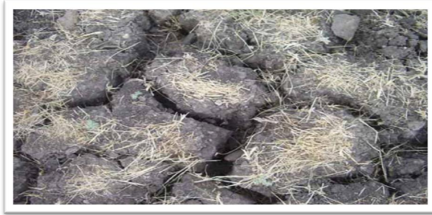
Figure 1.1 Typical Expansive Soil with Polygonal Cracks
