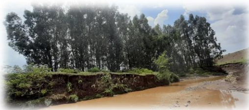
The bank instability of sampling site 5
