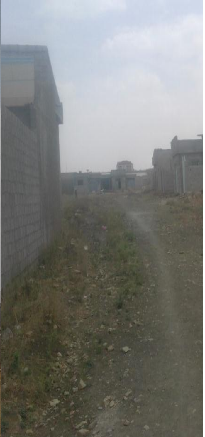
Figure 10: The unpaved road surface Source: own field Photo, 2018
